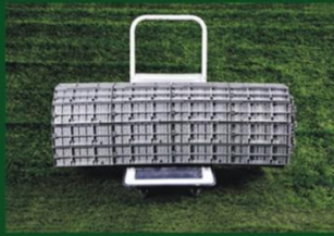
1. Take flooring to turf by little handcart or fork truck
